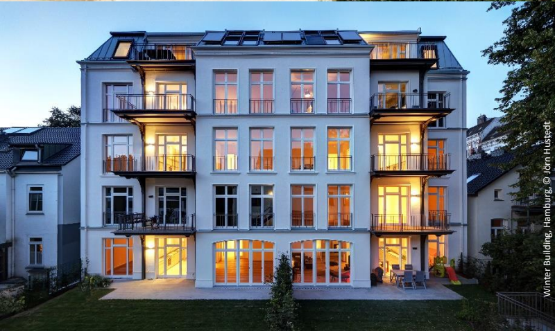
Passivhaus in Kassel, Stern Hermines
